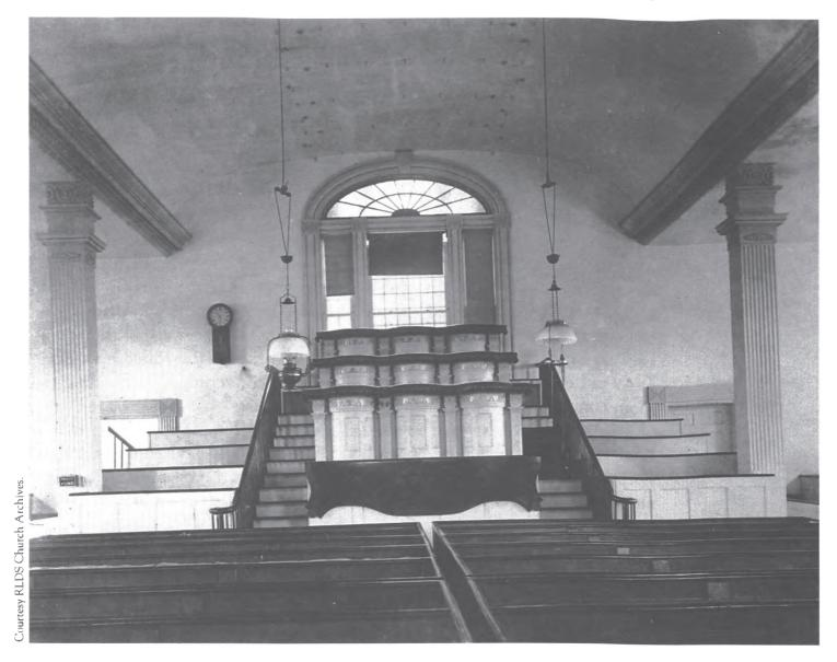
6-2. Lower court, east pulpits and window, showing hooks in the ceiling above the pulpit. These hooks, which were removed before 1934, supported the curtains, or "vails," that could enclose each tier of pulpits. A four-inch space between the two sets of center pews served as a passage for one of the curtains dividing the congregational space. Photographed about 1888.
