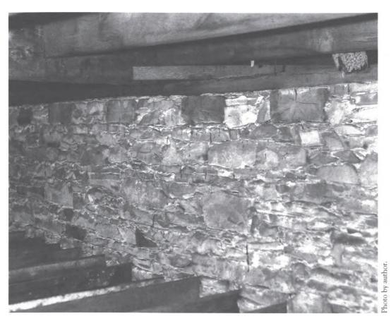
4-3. Masonry wall above the upper-court ceiling and below the attic-office floor, one of the few places in the temple where the roughly shaped sandstone blocks can be seen.
