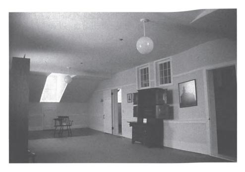
**4-7.** Western office used by Joseph Smith, Kirtland Temple. The doors and windows on the interior wall are placed between the posts and diagonals of the roof truss.
