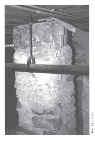
Fig 3-11. Detail of unused masonry pier directly under the window in the center of the vestibule wall. There is no physical connection between the pier and the girder above. Also visible are the large cast-iron pipe of the sprinkler system and smaller conduit carrying electric wiring.
