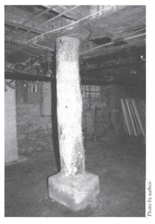
Fig 3-4. Timber prop supporting the lower-court floor girders at midspan. Note that the foundation of the timber prop is merely a block set on the dirt floor. In addition to the piping, wiring, and conduit visible in the photograph, a paint spot on the wooden girder identifies a surveying point which is checked periodically to ensure that these provisional repairs are not settling on the dirt floor.
