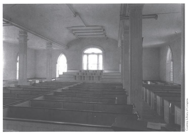
6-8. Upper court, facing west, Kirtland Temple. Photographed April 1934 by Carl F. Waite. The rollers set against the ceiling were designed to carry canvas curtains that would divide the congregation's space into four separate rooms and and would partition the multiple pulpits into separate worship spaces. Note the slit in the elliptical arch, just visible in the
