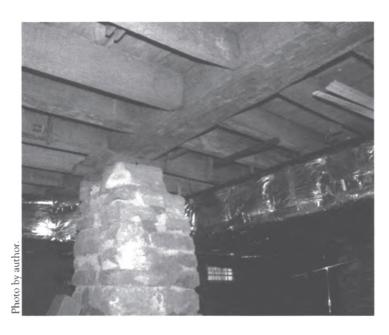
Fig 3-3. Detail of girder and pier supporting floor of lower court. Also visible are the masonry pier supporting the girder and joists framing into the girder. Modern additions include the insulated ductwork.
