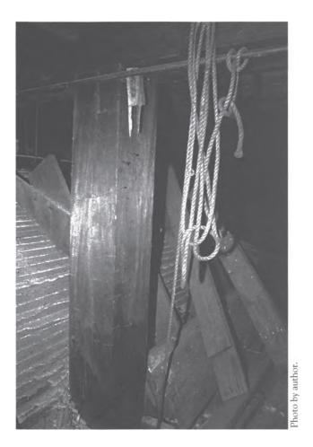
6-4. Detail of broken remnant of pulley carrier above the upper court. The rope is attached to the drum and crank below for illustrative purposes. Note the wrought iron cut nails still imbedded in the column after the pulley carrier split and broke away.
