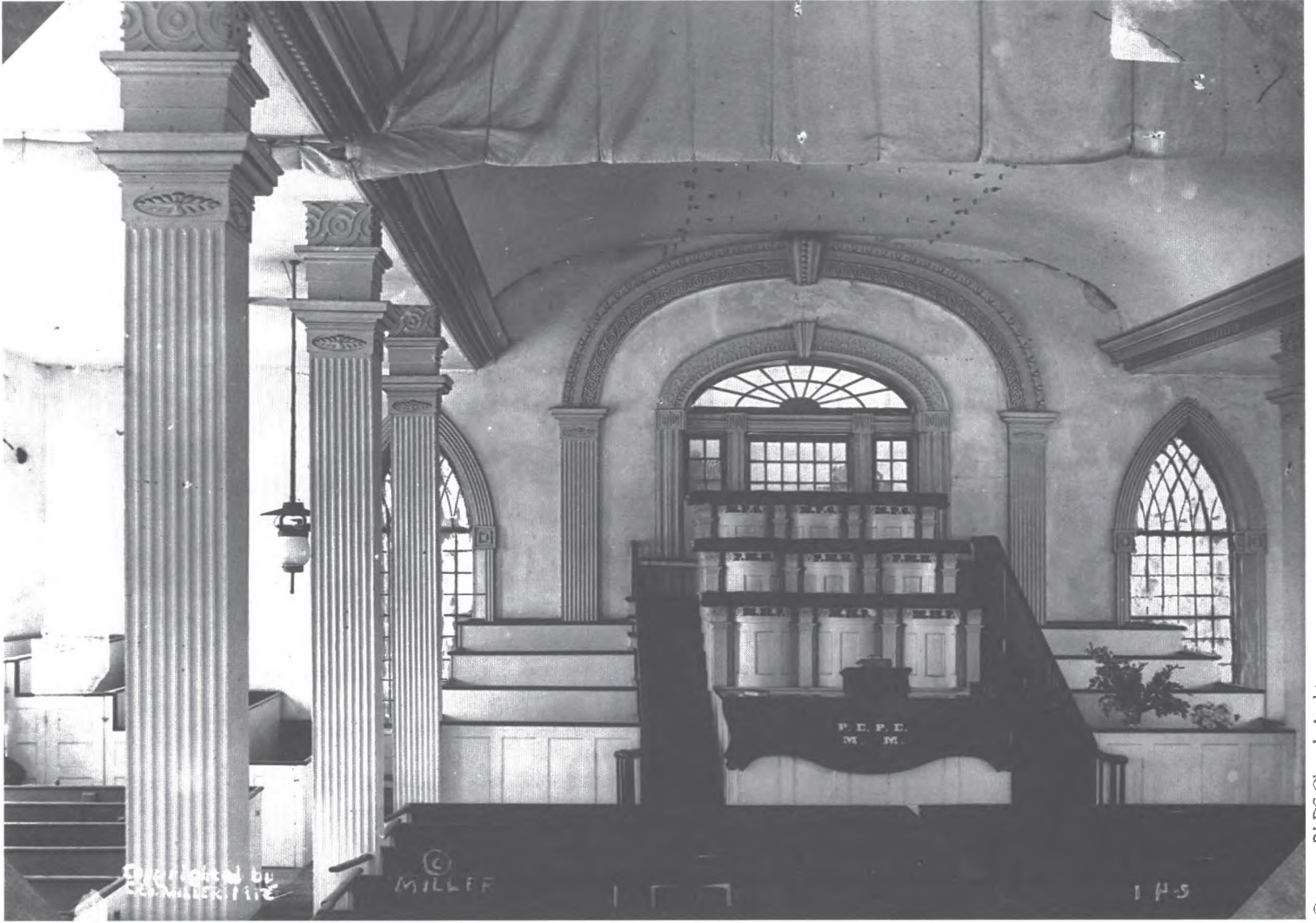
6-1. View of curtain in lower court as seen from the east, Kirtland Temple. Although the curtain was part of an 1887 replacement system, the photograph shows how the original curtains
