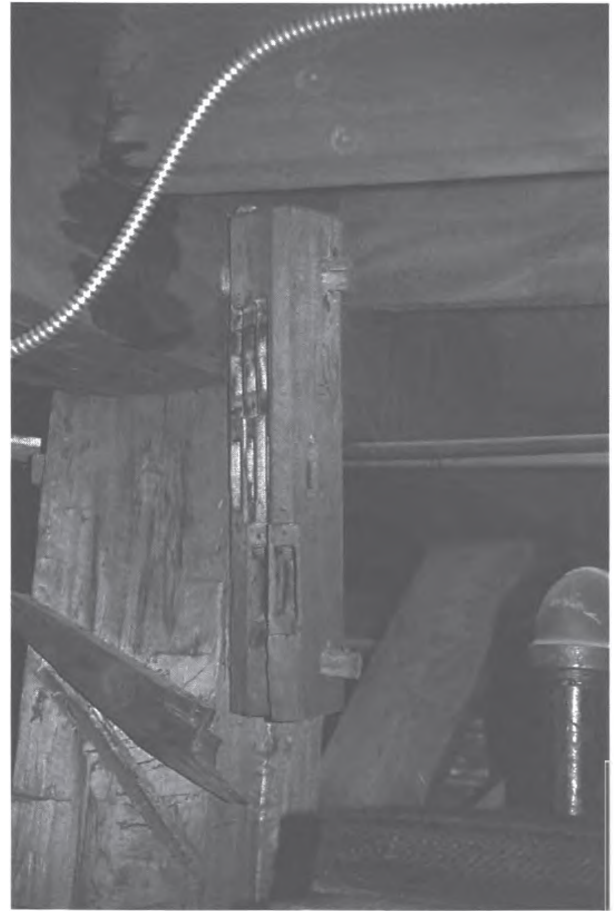
6-5. Detail of pulley carrier above the lower court. Note the wooden pegs used to attach the carrier to the wooden column.
