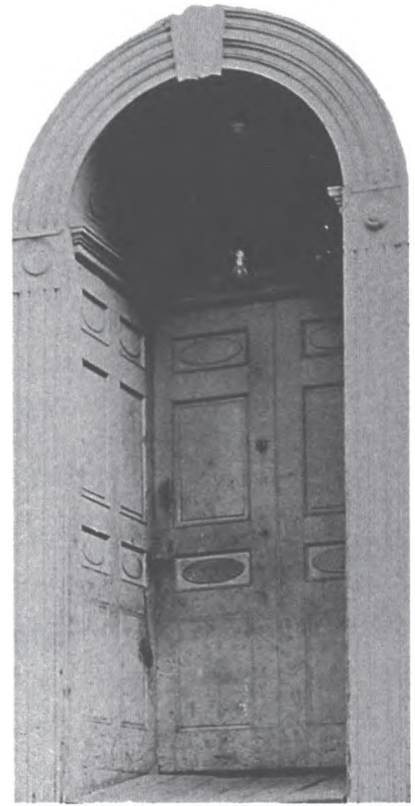
4-2. Detail of entrance door, L'Assomption, Quebec, from Frary, Early American Doorways , 1937. Note the raised elliptical panels.
