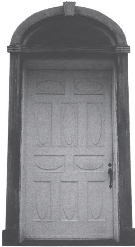
4-1. Raised elliptical panels on entrance door, Kirtland Temple. Elliptical panels are a feature found in Canada (fig. 4-2) but not in Ohio or New England. Photo by author.
