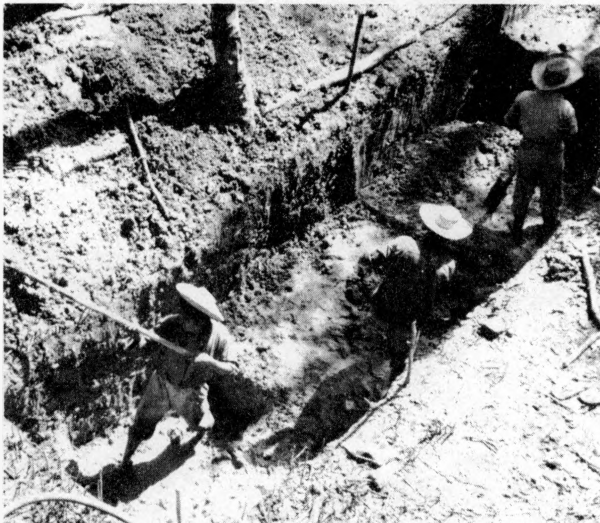
Digging the sump in Mound E-3.
