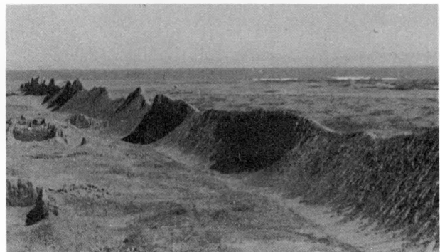
The northwest wall of the Cabildo or Labyrinth compound at the ruins of Chanchan, near Trujillo, looking westward toward the Pacific Ocean. Chanchan was once the capital of the Kingdom of Chimor.
