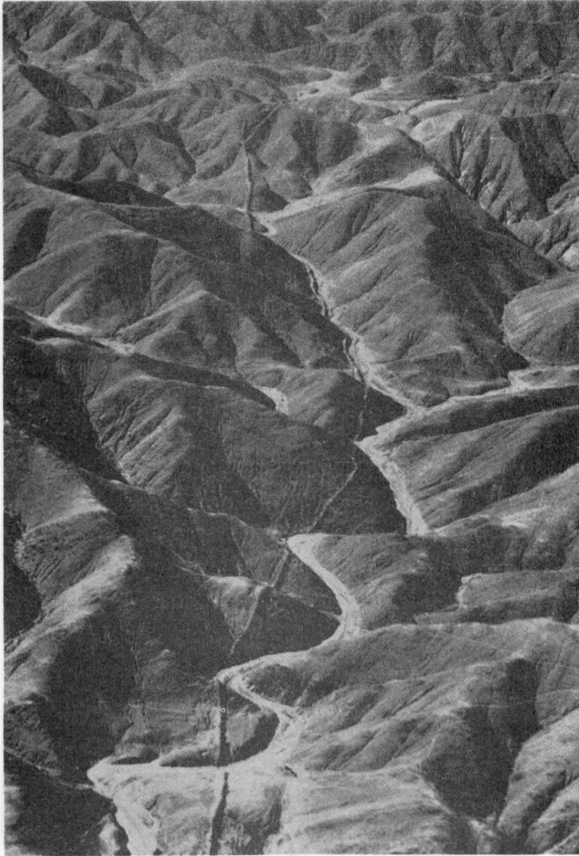
The "Great Wall" of Peru. This enormous structure begins just north of Chimbote and runs for more than 40 miles inland across the mountain spurs which line the northern edge of the Santa River valley. Here the wall is seen crossing a tributary. Photo by Lt. George R. Johnson.
