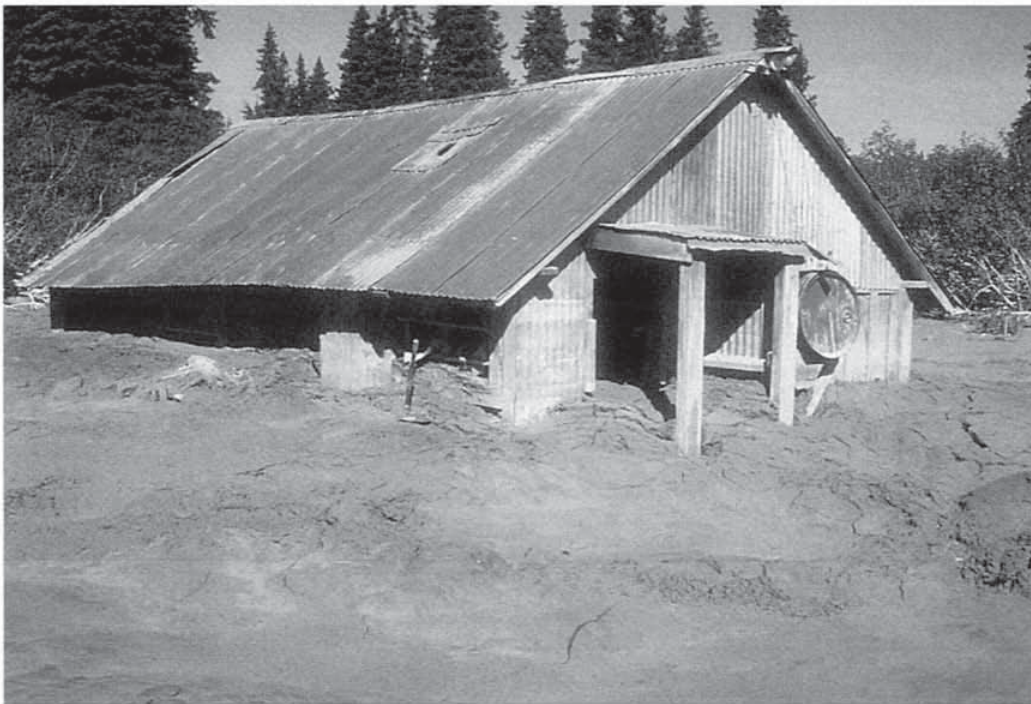
Building buried by lahars (volcanic mudflows), 1990. This structure, located near the mouth of the Drift River in Alaska, is twenty-two miles from Redoubt Volcano, the source of the eruption. Photograph by C. Gardner. Courtesy USGS.
